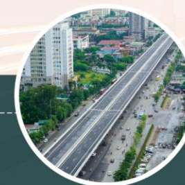
Basic completion of Ring Road 3 (Hanoi)
