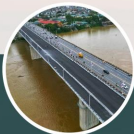
Completion of Vinh Tuy 1 Bridge (Hanoi)
